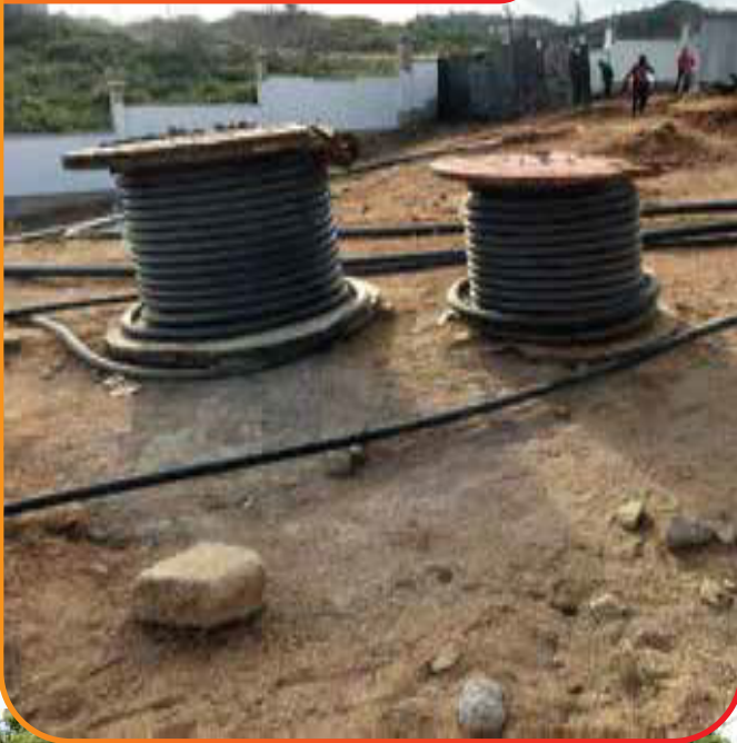
240mm 2 XLPE /PVC/ CU/ Cable Electric Installation
