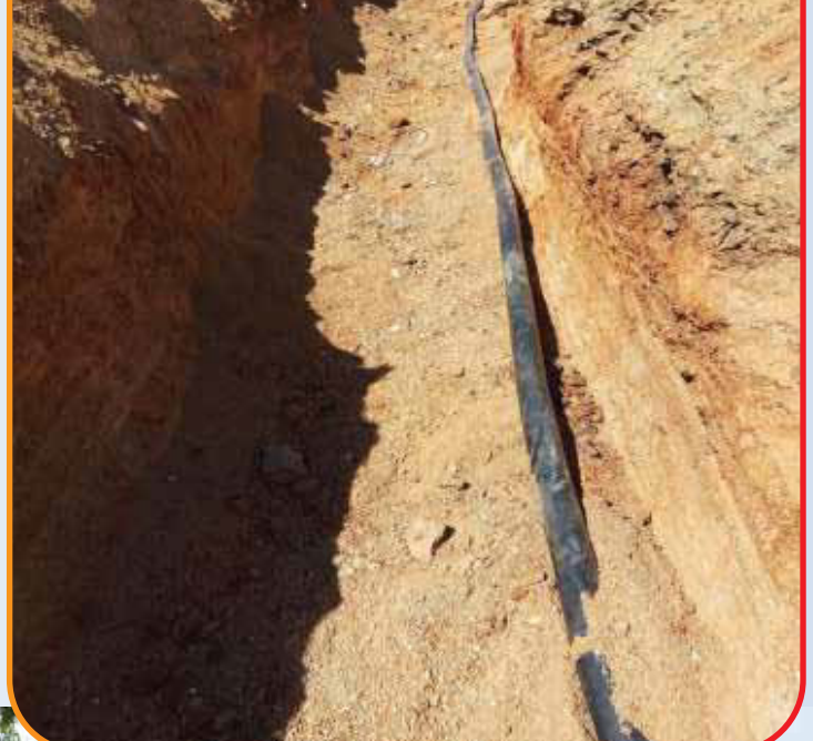
Laying of 240mm 2 XLPE /PVC/ CU/ Cable Electric Installation
